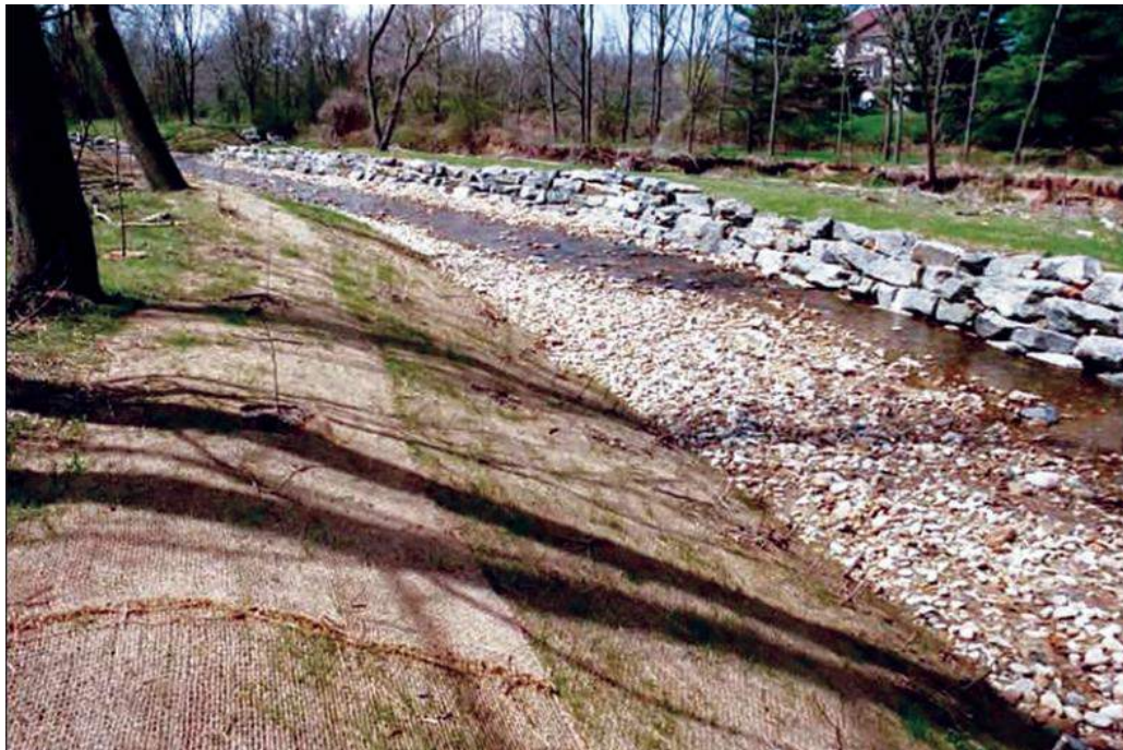
FIGURE 4. Restored section of Minebank Run (2005). View looking upstream from the confluence with the Harts Run tributary at the upstream end of the study reach with the original channel visible in the background. Image courtesy of U.S. Geological Survey Scientific Investigations Report 2012-5012.
